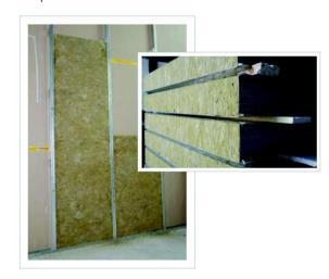
Before installing TUFFINSUL Rigid Slabs, make sure to clear away any dust or grease and dry the surface. Slabs are pre-cut in required dimensions and placed over the surface to be insulated. Care should be taken to ensure that the joints fit property and no gaps are left at the jobs. Depending on the surface and equipment. pins or spacers should be used to fix the Slabs in place.
